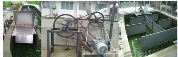
Figure 3. Paddlewheel and pulley system of the open raceway ponds.
