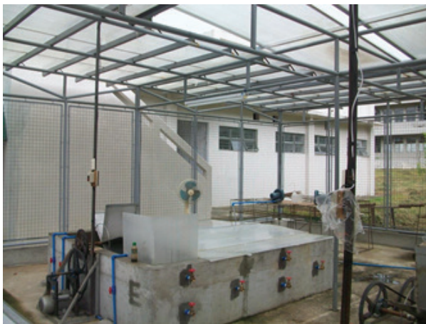
Figure 7. Sampling ports of the multi-stage open raceway pond at different heights.
